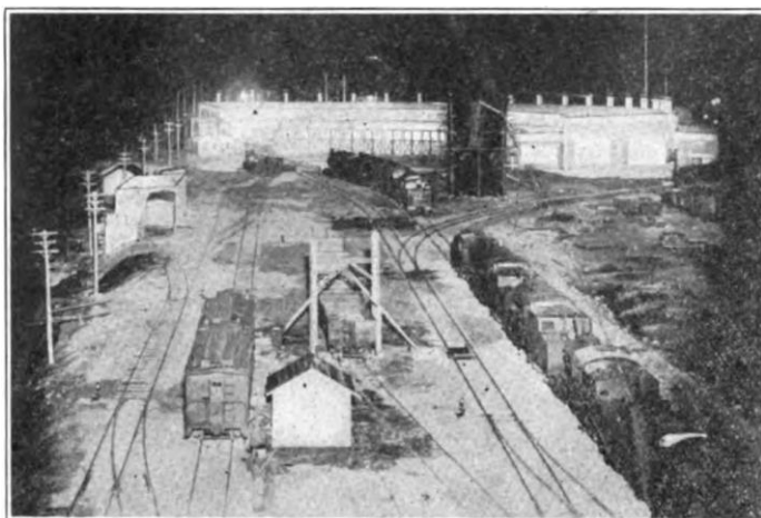
Night View of Toledo & Ohio Central Engine Terminal, Columbus, O.
